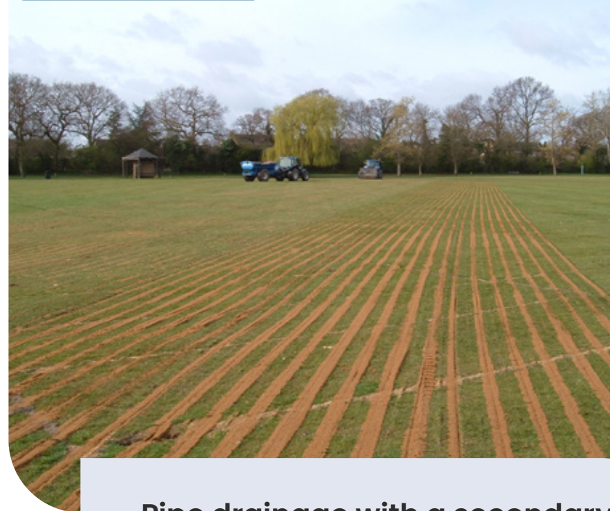
Sand grooves installed at 260 mm centres
