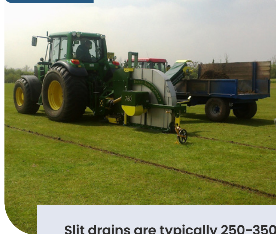
Installation of slit drains in progress
