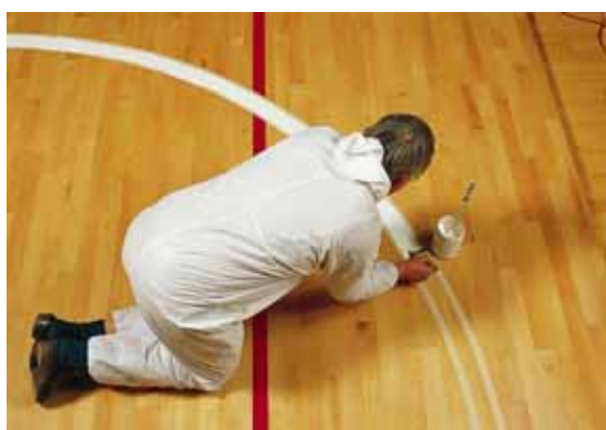
Painted line markings.
