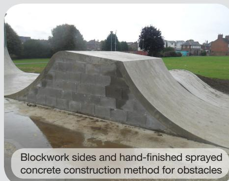
Blockwork sides and hand-finished sprayed concrete construction method for obstacles
