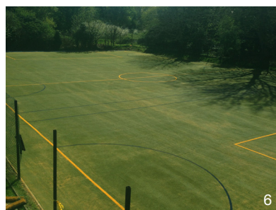
Recycled carpet installed onto a block of macadam surfaced tennis courts to create an artificial grass pitch
