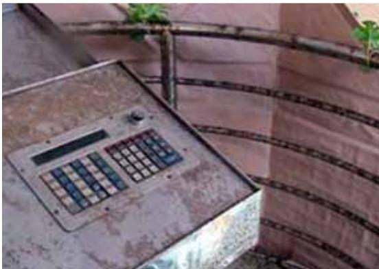
Corrosion of stainless steel balustrading and control panel exposed to pool atmosphere
