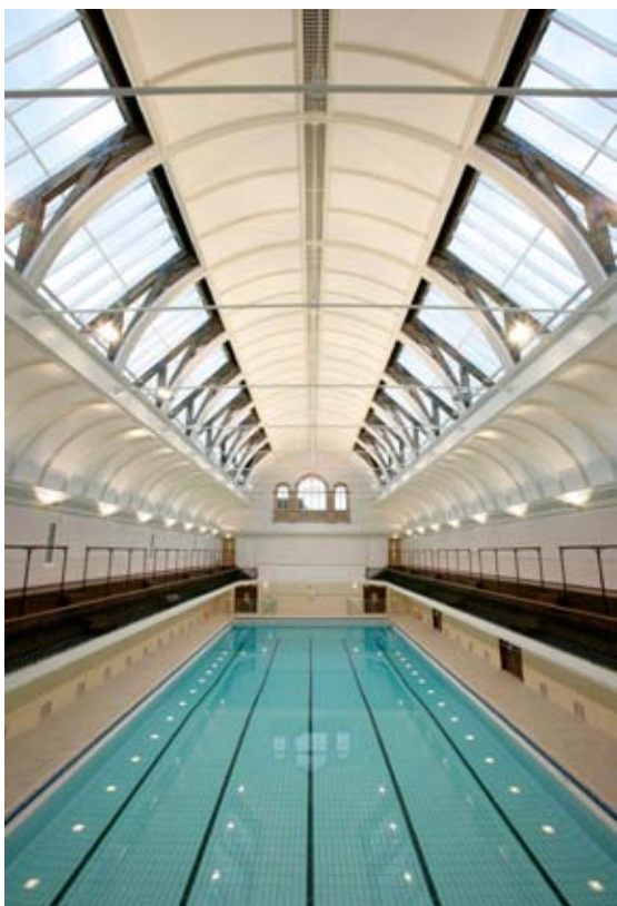
Historic renovation together with sensitive upgrade to meet current standards
